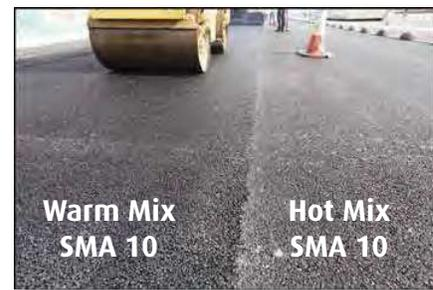
**Figure 7** Surface texture of both warm and hot mix SMA 10
