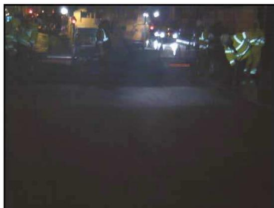
While it took a couple of batches for the plant operator to bring the mixing temperature down to the target of 30°C less than that of the hot mix, once the lower temperature was achieved it was easily maintained. Onsite, the laying crew reported that the material behaved in the same way as conventional hot mix. Images from the thermal imaging camera showed that the mix temperatures were consistent at about 30°C lower than the hot mix, as can be seen from Figures 1 and 2 above.
