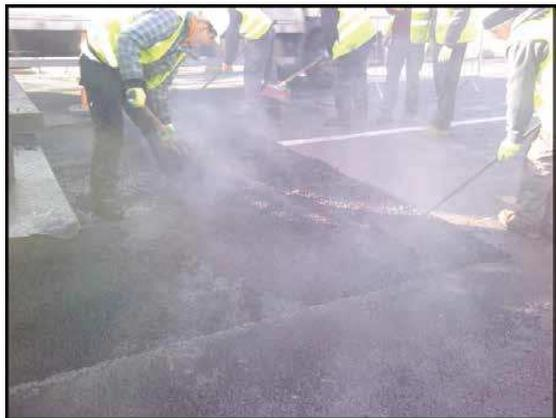
Figure 5 Smoke from hot mix SMA 10
